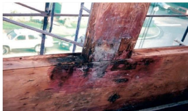
Figure 1 – Damage to wood rough opening, resulting from moisture accumulation
